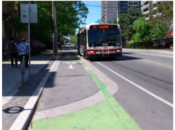
Figure 10 - Curbside Raised Cycle Lane
