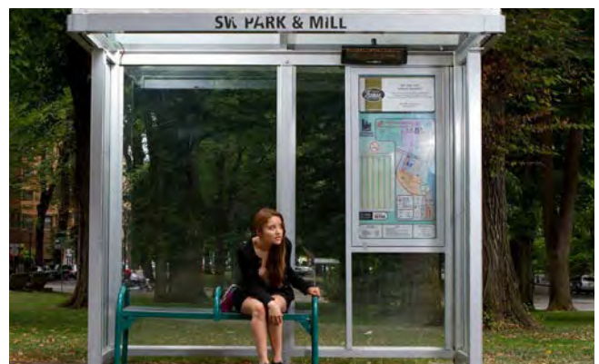
Open shelter for ease of seeing approaching bus
